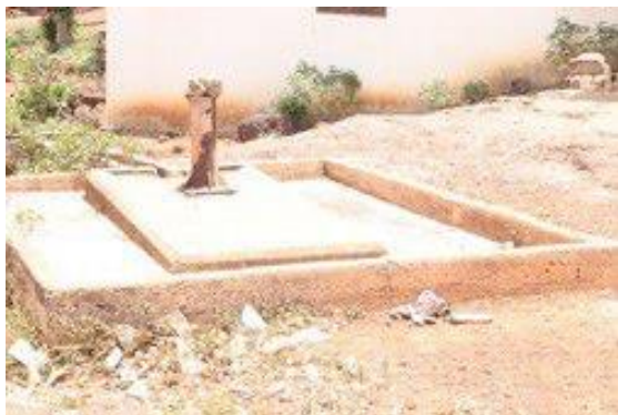
Image 1. Hand pump well in need of rehabilitation
