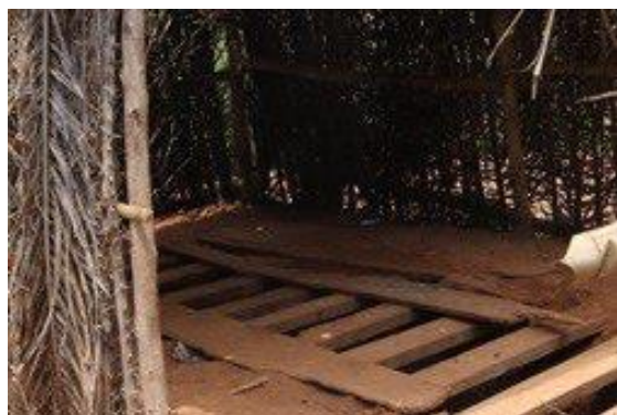
Image 5. Existing toilet facility made of wooden slabs over a pit
